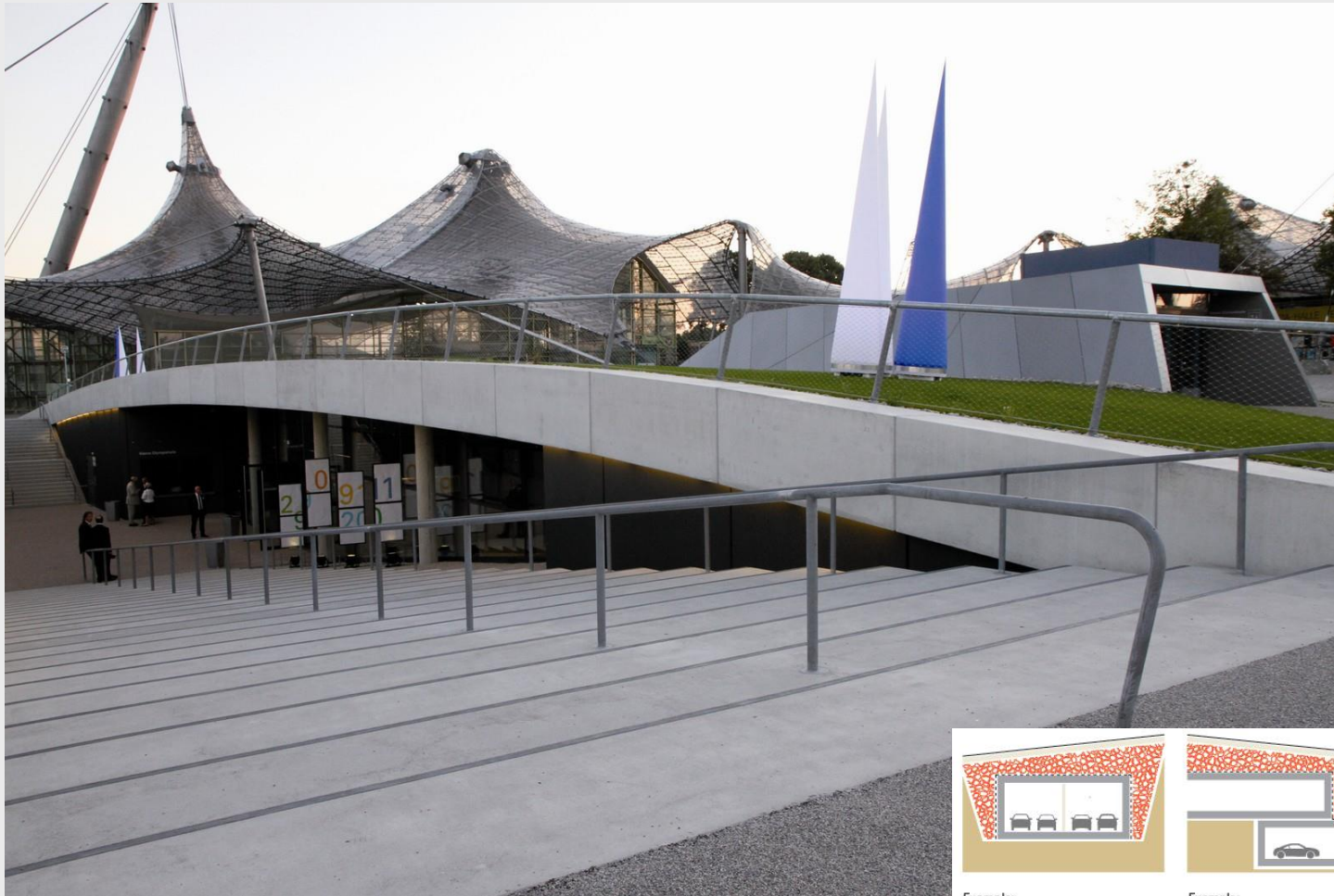
Small Olympia Hall in Munich, Lightweight infill 800 m 3 Cellular Glass Gravel
