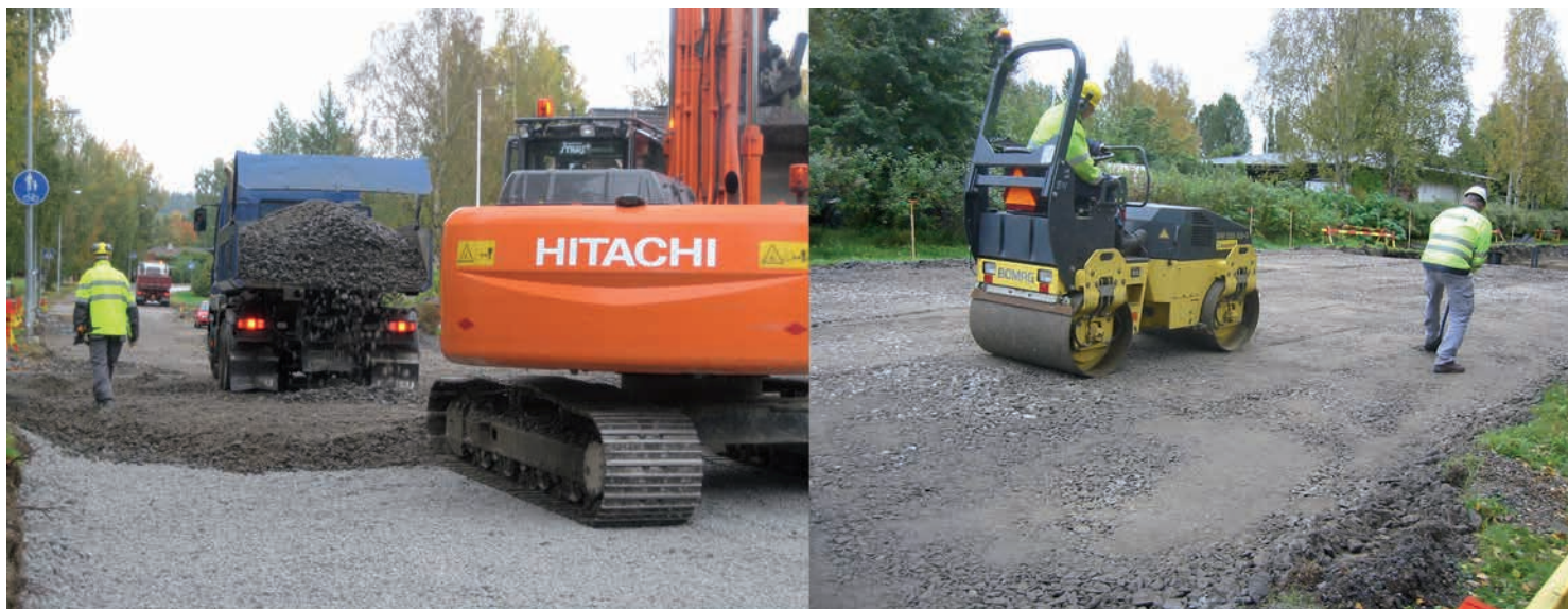
Figure 10. The final compaction over a 150-200mm layer of mineral aggregate.
