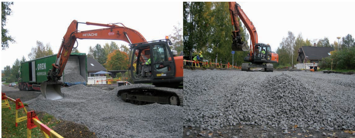
Figure 9. The unloading of foamed glass aggregate from the delivery vehicle as well as the spreading and pre-compaction of the material.
