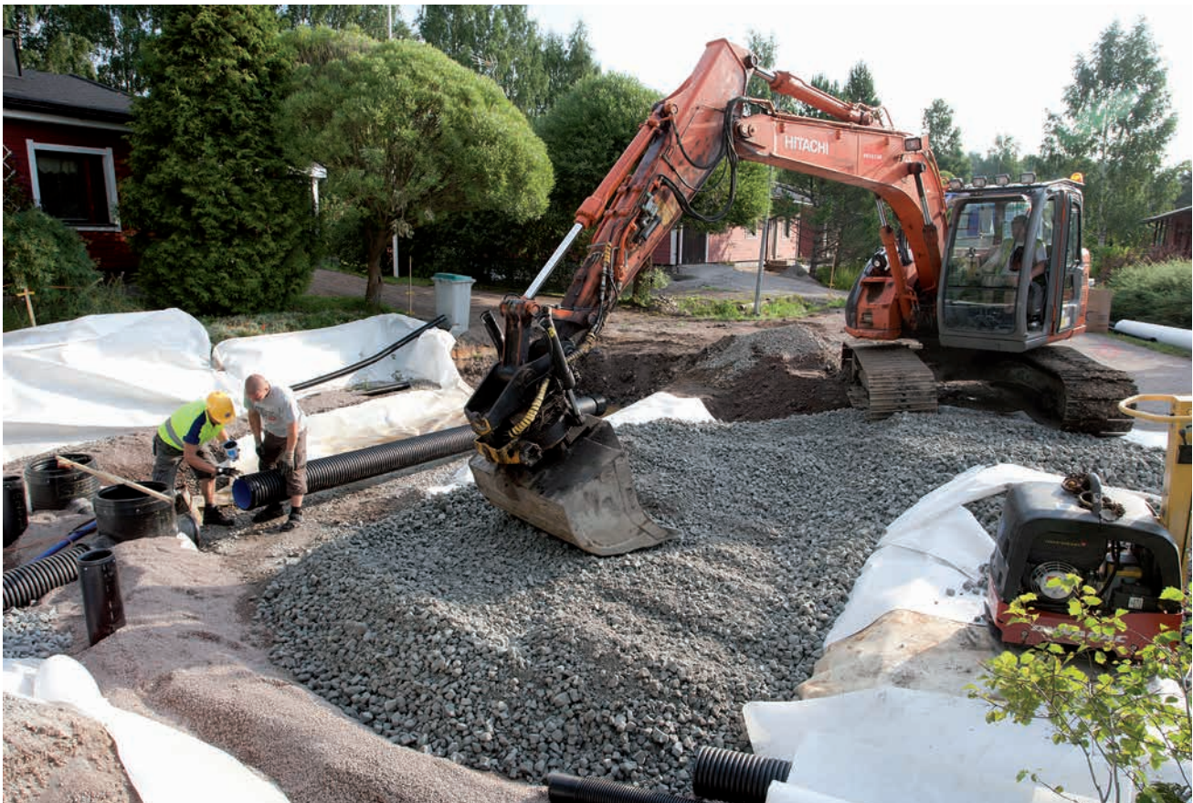
Figure 1. Foamed glass being spread on a worksite
