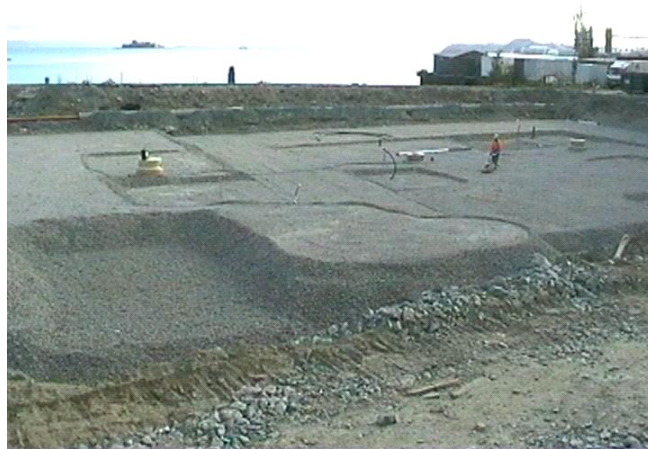
Figure 6: Foamglass LWA used as a lightweight fill material, building in Trondheim
