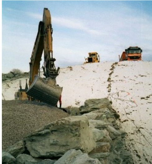
Figure 7: Foamglass used in project E6 Eggemarka as light weight fill material
