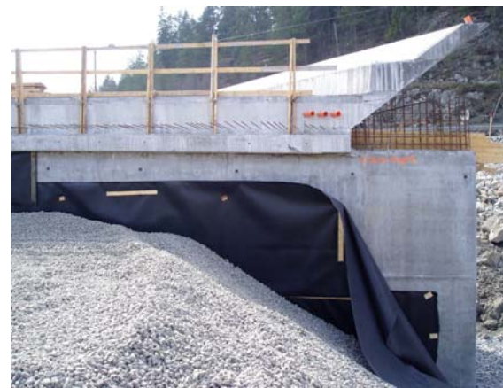
Figure 3: Road E6 at Klemetsrud. Foamglass as light weight material
