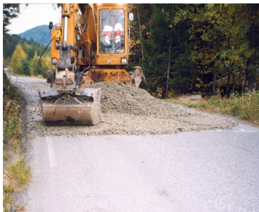
Figure 2: Foamglass used as insulation material
