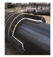
system; more pieces/parts means more seams and joints to seal, which means more labor, more consumption of materials, and more possibility of improper installation (e.g. a seam not sealed, or a cracked piece of insulation) - - which can lead to thermal and/or moisture leaks; a cellular glass insulation system is also likely to have more layers than a comparable phenolic system thus requiring more steps in the process,
