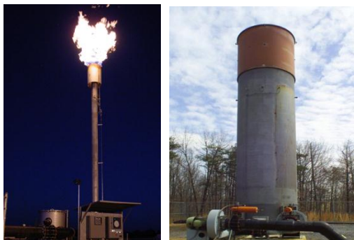
Figure 1-4. Open (left) and Enclosed (right) Flares
