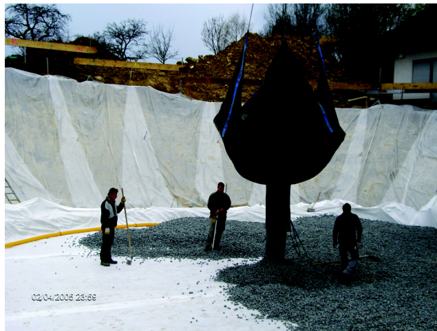
Figure 8 Placement of cellular glass aggregate with the help of a crane and a sheet with a plug valve onto which the cellular glass is unloaded from the truck. (Reproduced by permission of Misapor AG.)
