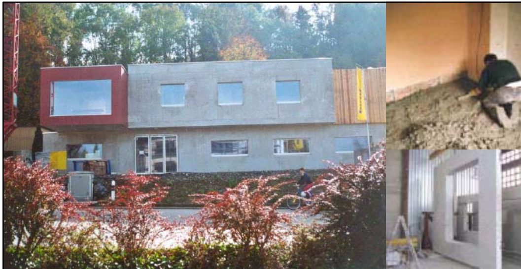
Figure 11 - A concrete building built using Misapor lightweight concrete.
