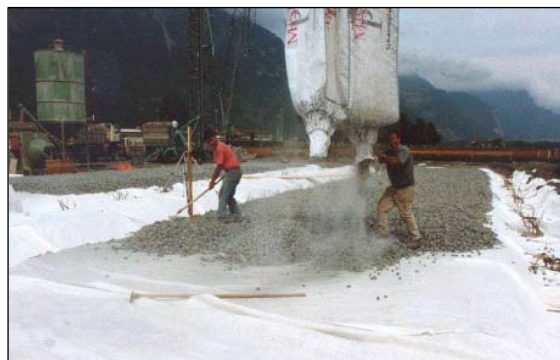
Figures 7 and 8 - Foam glass exiting the furnace and being used for a loose aggregate floor insulation
